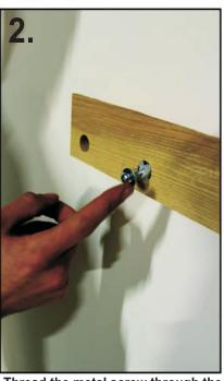
Thread the metal screw through the plastic washer until it threads till the wall
