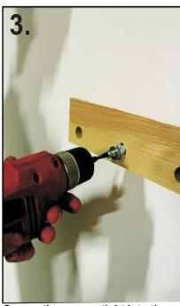
Secure the screws tight into the hole drilled in the wall with the help of drill
